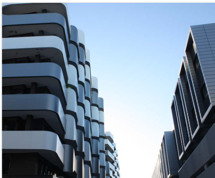
Tip Top Building (Melbourne, Australia)
